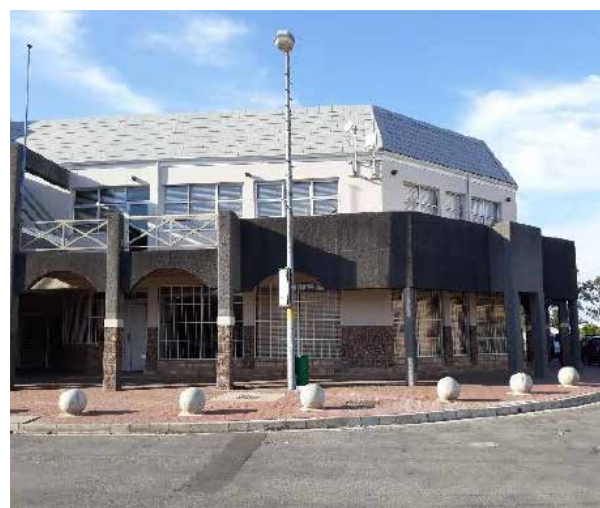
Bisho building after redevelopment
