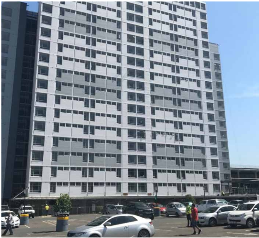
Malvern Heights after redevelopment
