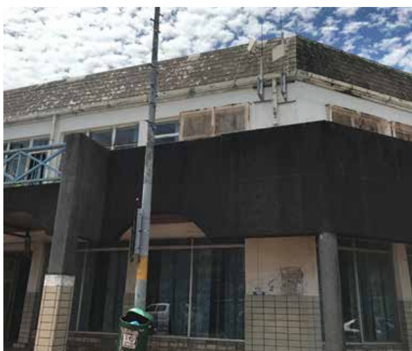
Bisho building before redevelopment
